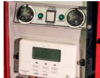
The control panel is housed behind the large, left door.
